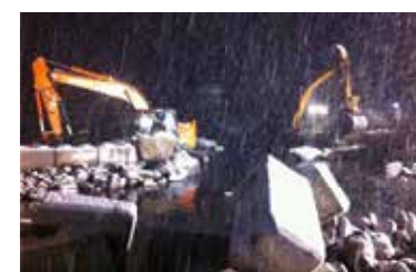
Oben: Wave Testing Grounds at low flow. Unten: Midnight berm construction in blizzard.
